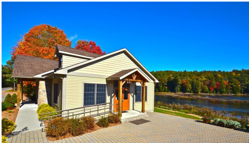
Bolton Community Center at Bolton Conservation Park
