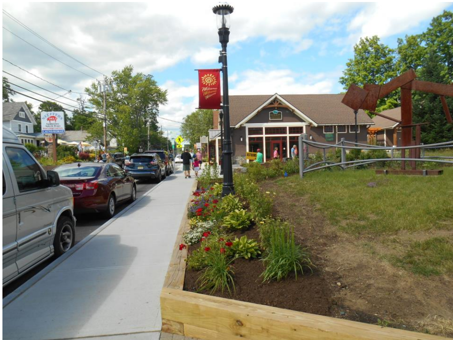
Bolton Landing Streetscape
