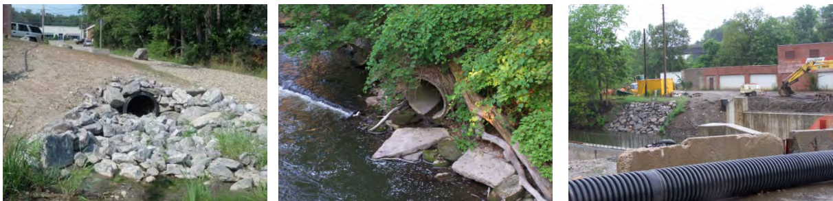
(Left) Stone riprap at Clifton Avenue. (Center) Concrete rubble at Buffalo Street. (Right) Stone riprap at the Sprague Street Bridge.
