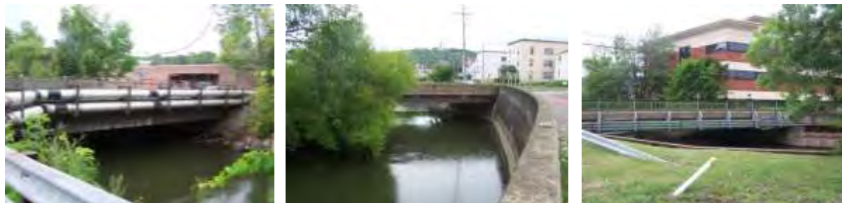
(Left) BPU District Heat piping hung on the north side of the Harrison Street Bridge near Institute Street. (Center) Institute Street Bridge. (Right) Utility lines hung on the side of the Foote Avenue Bridge.
