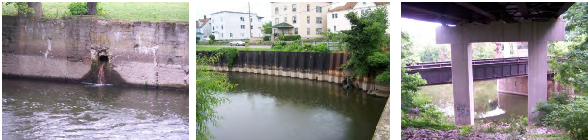
(Left) Concrete retaining wall below the Warner Dam. (Center) Sheet pile wall below the Institute Street Bridge. (Right) Riprap under the 6 th Street Bridge.
