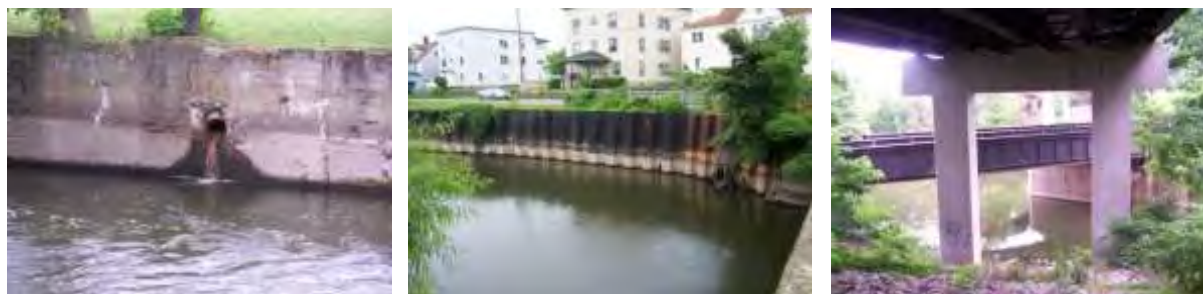
(Left) Concrete retaining wall below the Warner Dam. (Center) Sheet pile wall below the Institute Street Bridge. (Right) Riprap under the 6 th Street Bridge.
