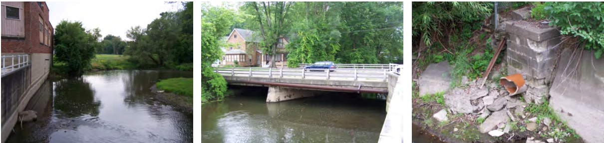
(Left) Concrete foundation wall on southern river bank. (Center) Utilities hung on the Hopkins Avenue Bridge. (Right) Stormwater discharge at southeast abutment of the Hopkins Avenue Bridge.
