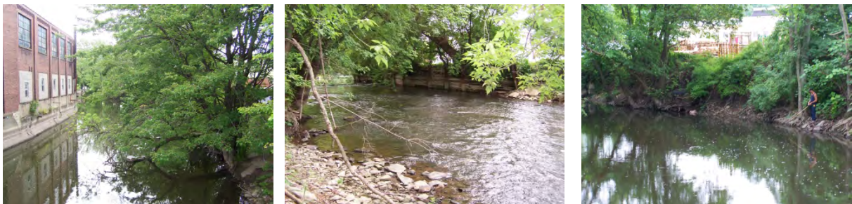
(Left) Riverside Industrial Center below the Foote Avenue Bridge. (Center) Steel pile and railroad tie armor off Allen Street and near River Street. (Right) Natural armor of roots below Hopkins Avenue Bridge.
