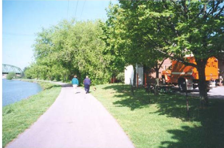
The village public works garage fronts on the canal. Options to lessen its visual impact on the canal should be explored.
