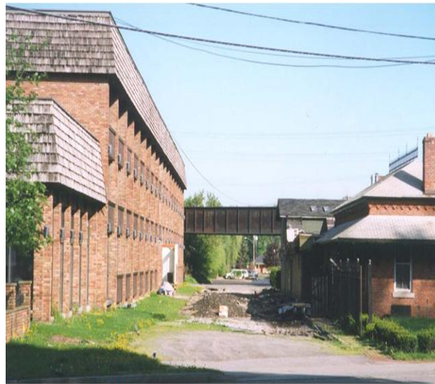
The former Depot Hotel, now the Depot Inn, is being converted to a luxury inn on the waterfront.
