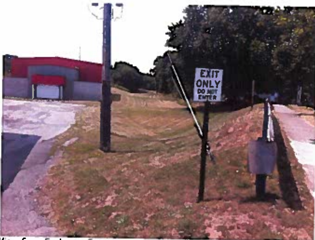
View from Exchange Street
