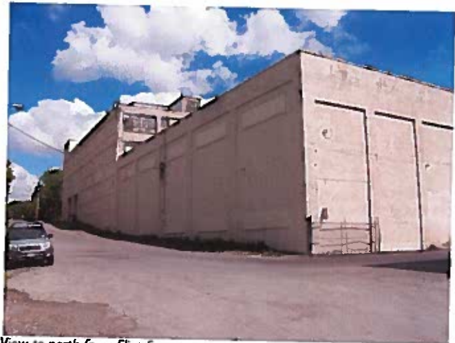
View to north from Flint St
