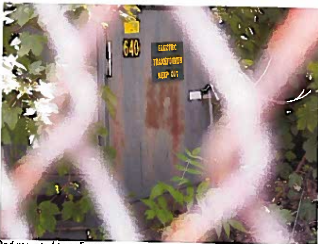
Pad-mounted transformer
