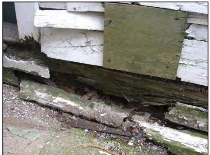
On heavy timber buildings, structural beams should remain covered and not be exposed to the weather.
