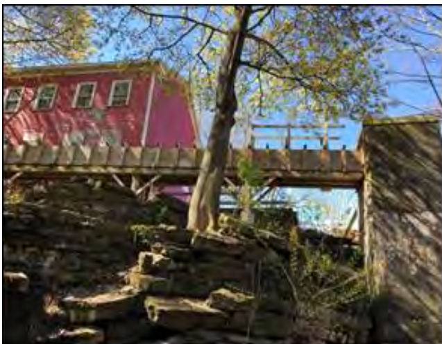
Figure 12: Reconstructed Raceway Structure for Mill
