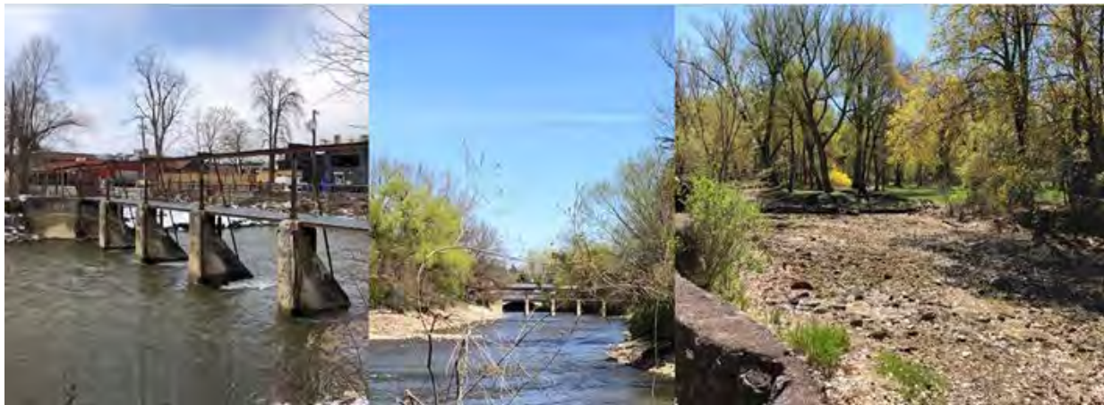
Figure 24: Island Park dam without the floodgates installed and the dry western creek bed
