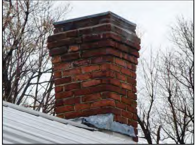
Chimneys and parapets should be inspected regularly for cracks and mortar integrity.
