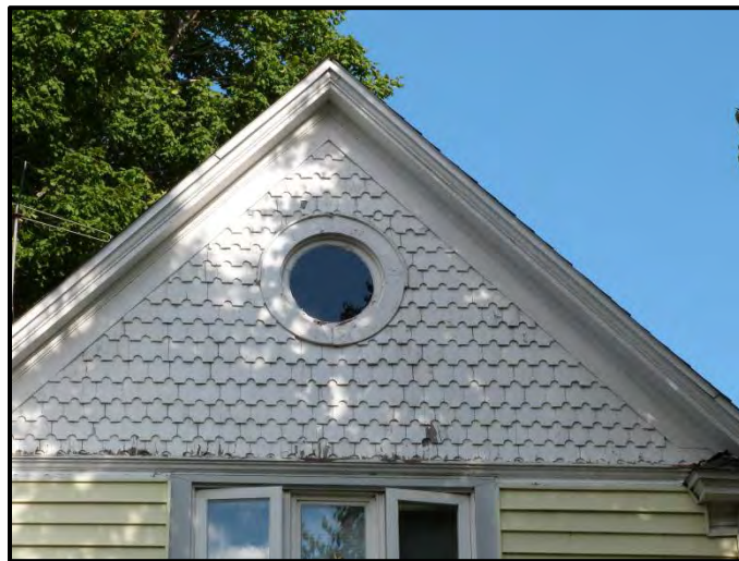
Decorative shingles and other similar features are often hidden beneath synthetic sidings added in later modifications.
