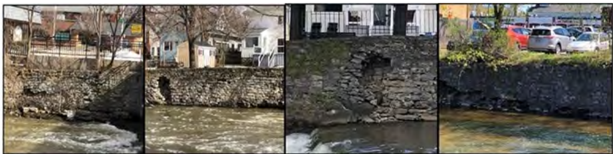
Figure 29: Photographs of structural deterioration of stone walls above Glen Falls
