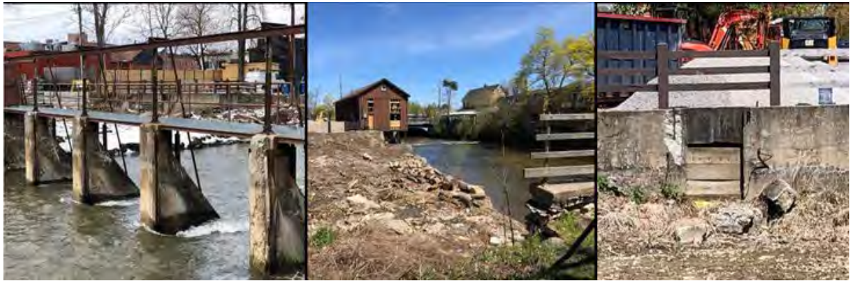
Figure 13: Deteriorating dam structure, deteriorated weir, and gate door for the Water Mill raceway
