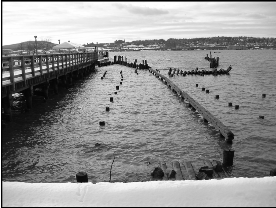
View looking down the north side of the new Newburgh-Beacon Ferry Pier at derelict pilings from the old ferry terminal. During low tide, all of these structures are visible; however during high tide, most of these structures are underwater creating an extremely dangerous navigation issue.
