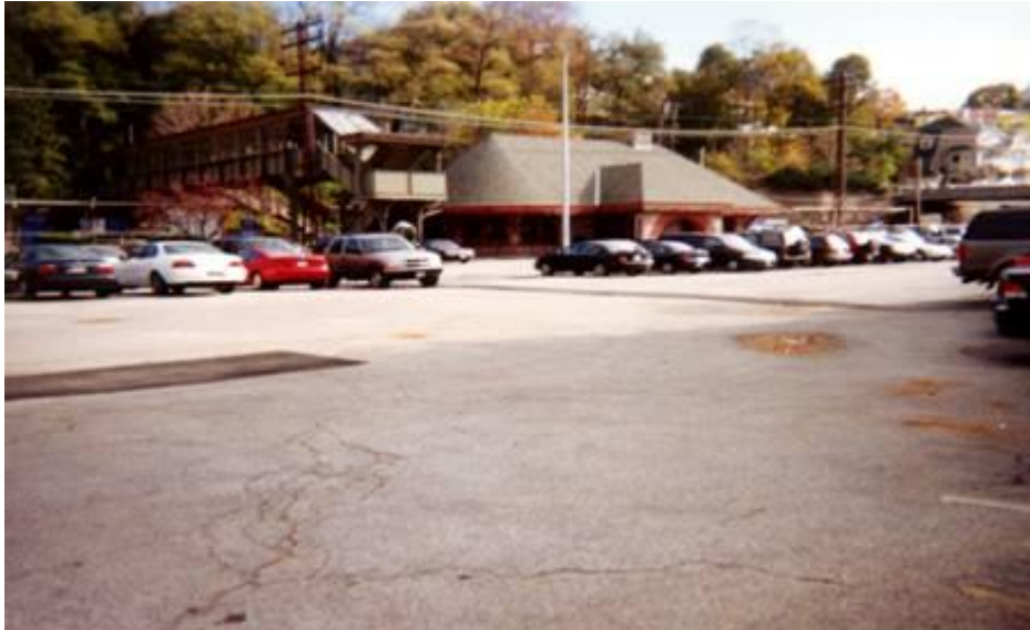
Photo 19 - Metro North Train Station
