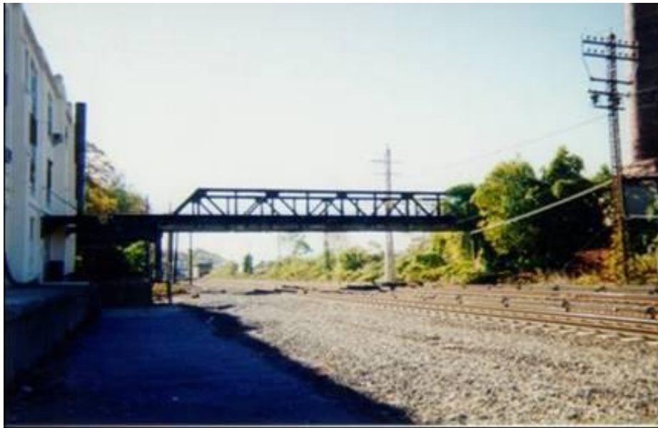
Photo 14 - Railroad Crossing at 145 Palisade (Bridge does not include sidewalks)
