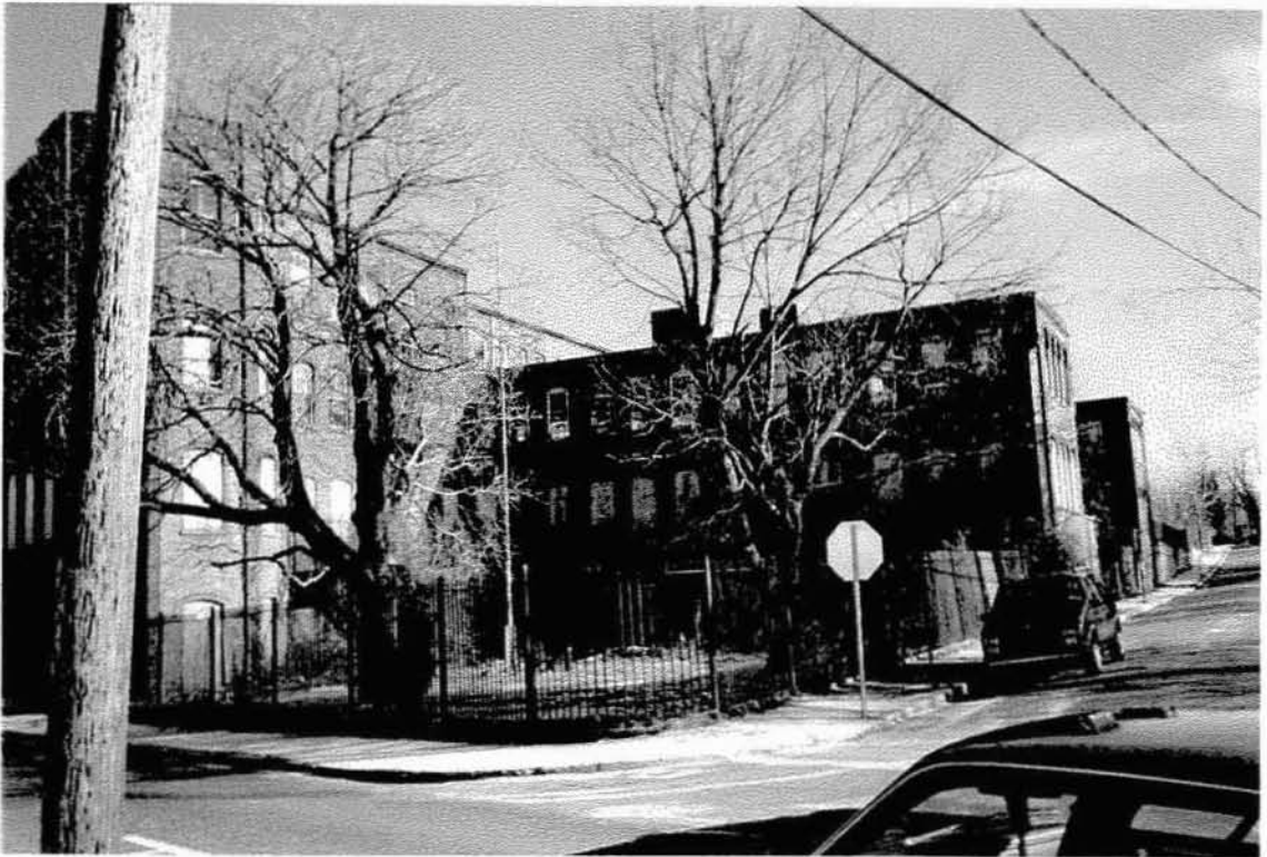
INDUSTRIAL CHARACTER AREA: Issue -- unused and decaying property
