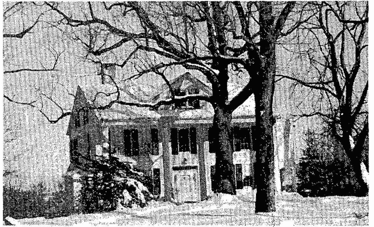
PHOTO #9: The "Bindery", the last industrial building ↘
