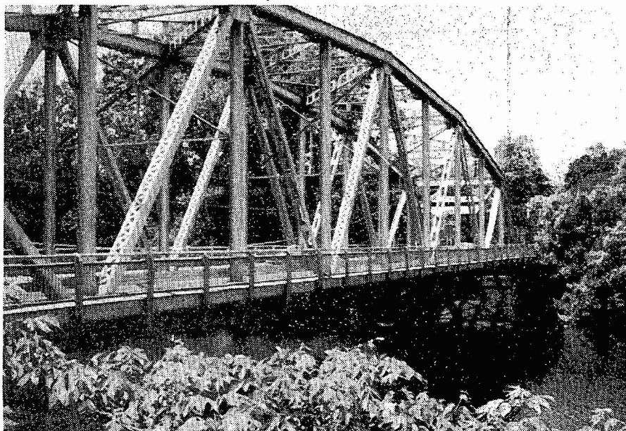
PHOTO #16: Steel bridge above the dam
