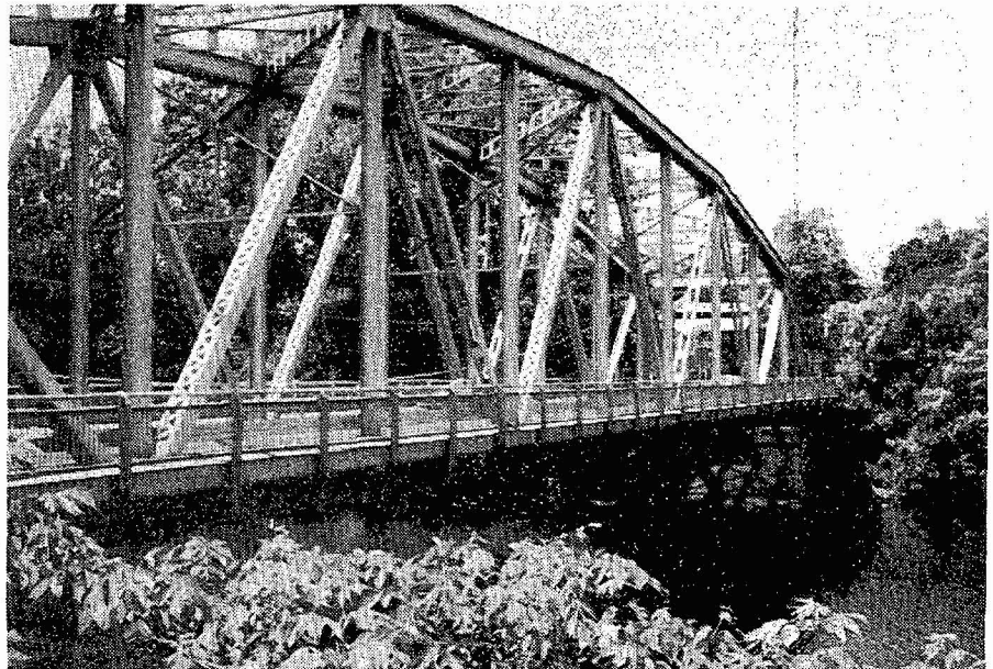
PHOTO #16: Steel bridge above the dam
