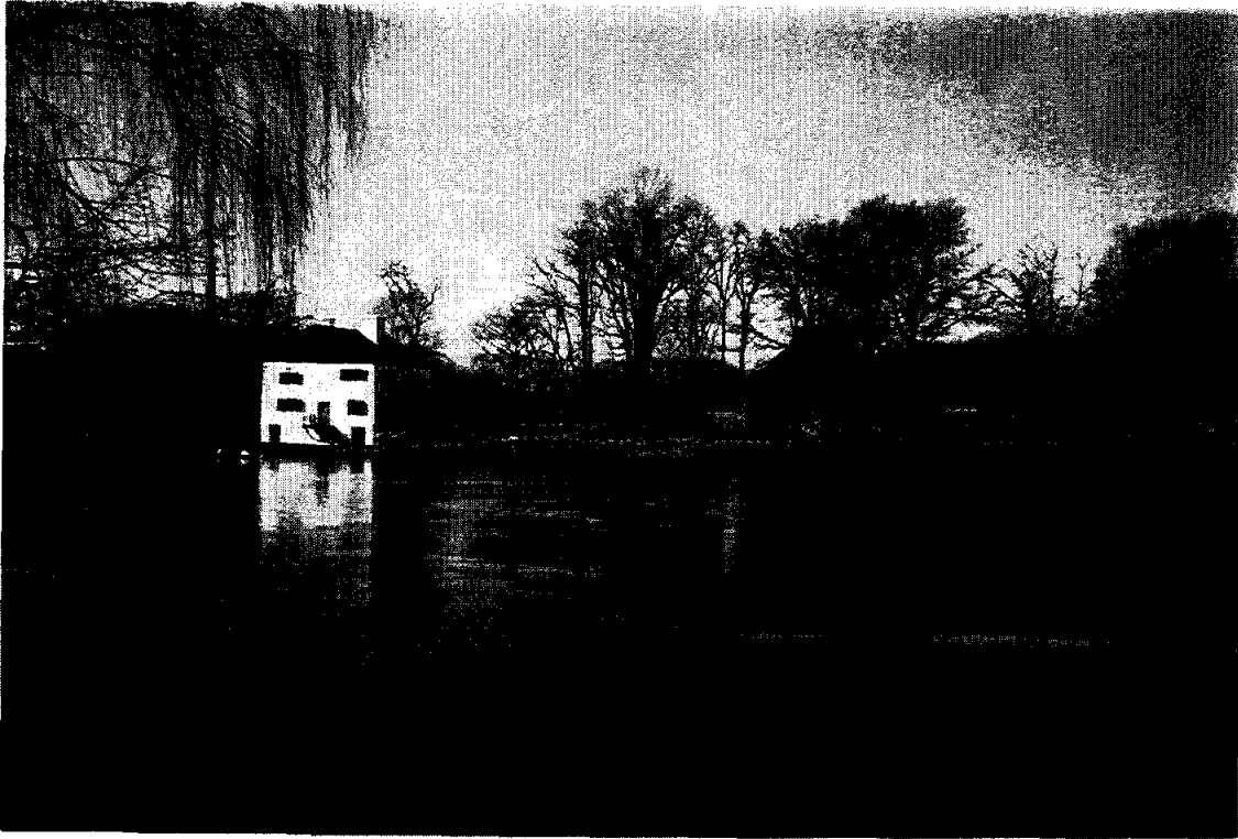
2 Philipsburg Manor Upper Mill Historical Site as viewed from U.S. Route 9 (North Broadway)
