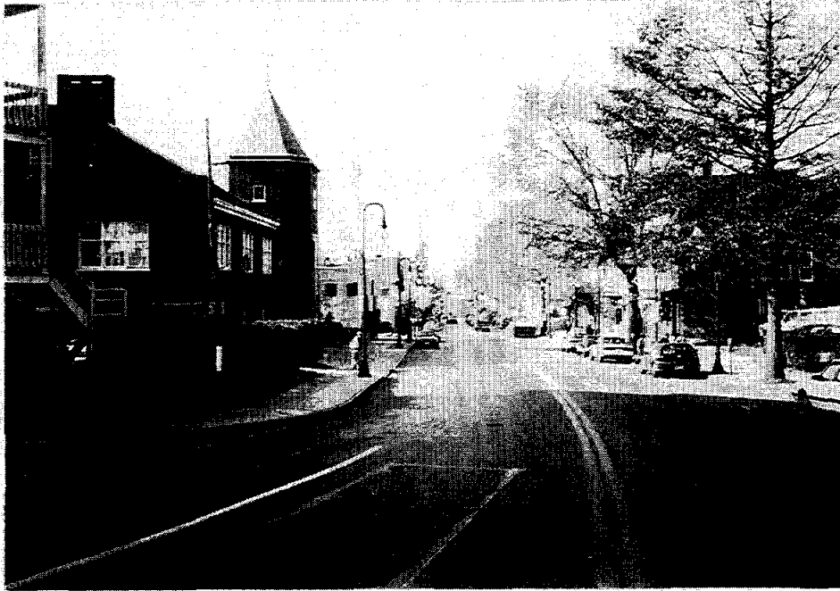
1 Beekman Avenue looking west toward Hudson River at intersection with U.S. Route 9 (Broadway)
