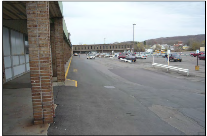
Binghamton Plaza parking lot has settled significantly causing a grade change between the building and support parking that makes full utilization of the facility challenging
