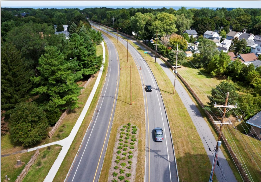
Seabreeze Drive in Irondequoit, NY was formerly NY 590 and underwent a transformation into a signature, multi-modal corridor complete with a green central median, multiuse trail and sidewalks.
