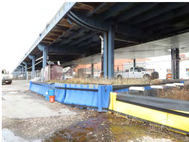
Pop-up wetland at Pier 5 capturing run-off from elevated I-87/MDE
