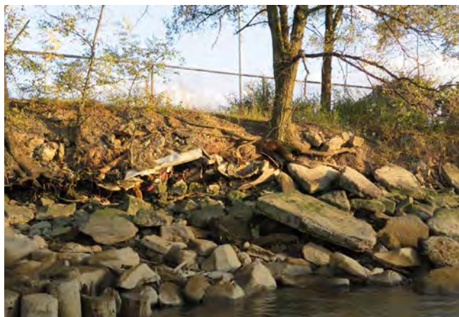
Stone rip-rap lines the banks of the Harlem River throughout most of the study area, with the occasional inclusion of a debris such as a junked car
