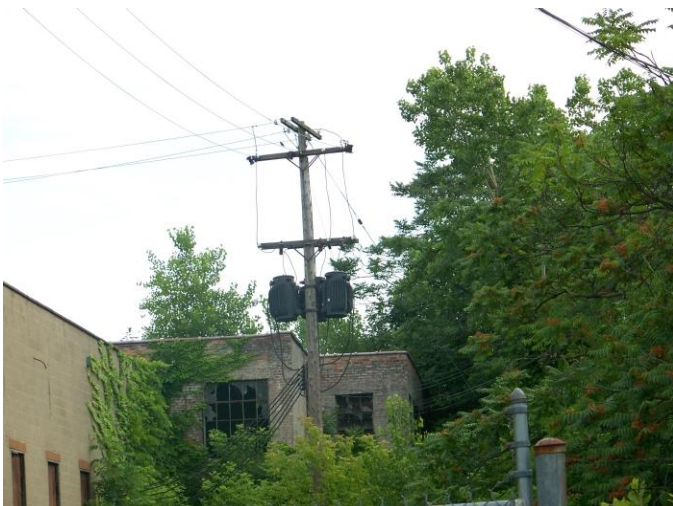
Pole-mounted transformers
