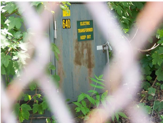
Pad-mounted transformer
