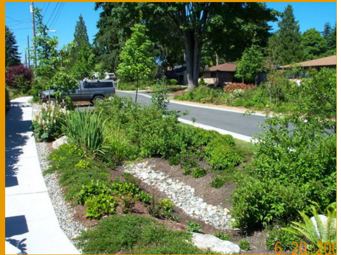
Residential Area Bioswale
