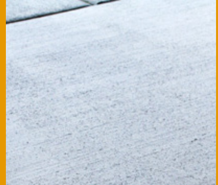
Broom Finished Concrete
