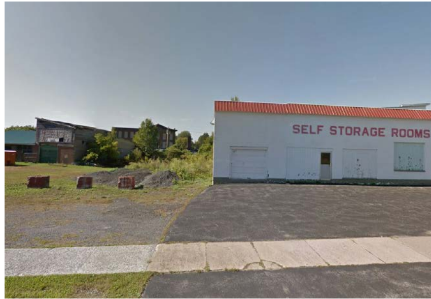
Current Building Conditions
