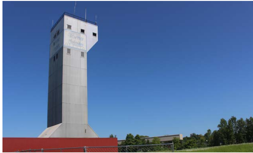
Existing Iconic Rome Tower Cable
