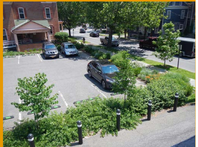
Bioretention and Pervious Pavement
