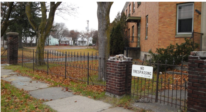
Portions of the City-owned structure, such as the brick columns surrounding the front of the building, are in need of significant repair.
